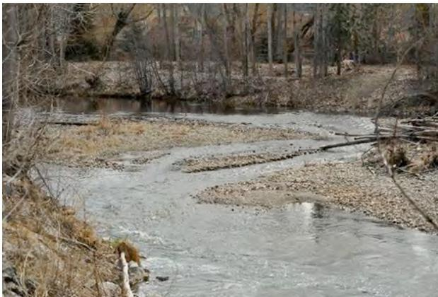
D5 - Riffle created to produce an upstream pond that feeds water into an irrigation ditch.
